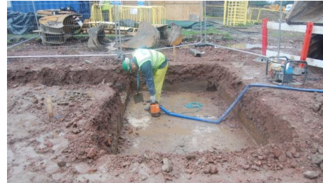
Figure 10: Pumping prior to Pouring
